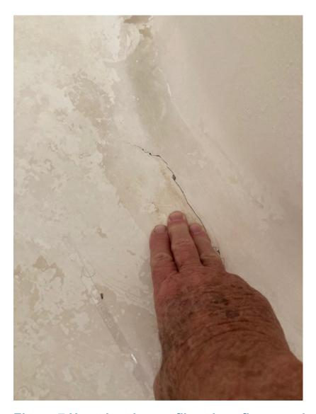
Figure 7 Upstairs shower fiberglass floor cracked water when showering has been leaking to ceiling in front room
