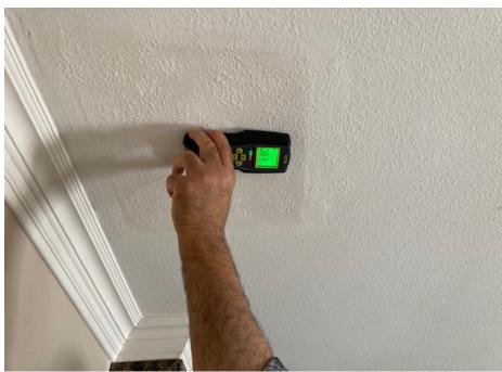
Figure 5 Just below toilet moisture from possible wax seal leaking
